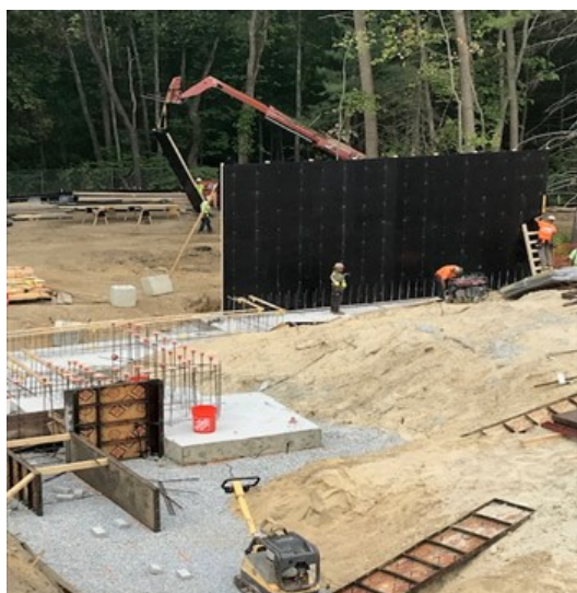
The first form for the lower level Foundation Wall August 17, 2020
