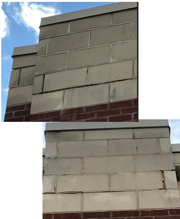
Failed mortar joints
