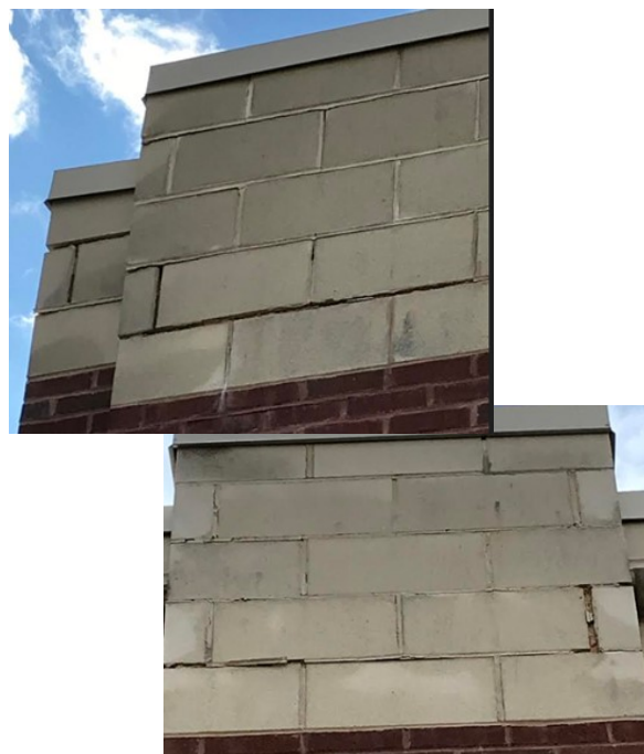
Failed mortar joints
