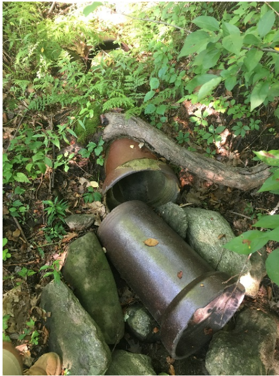
Tahattawan-2 Clay Pipe Outfall in need of repair
