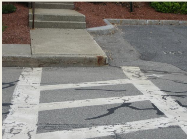
Mid-block crossing at the Sunny Delight Beverages Co. factory.
