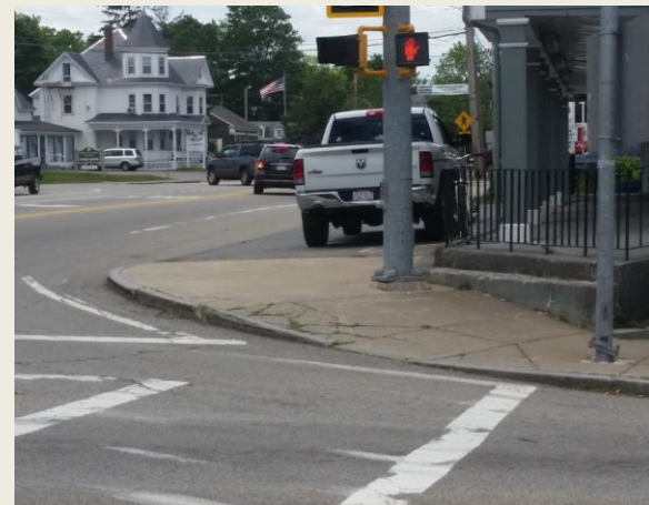
Southwest corner of the King St (Rt 2A/110) / Great Rd (Rt 2A/119) intersection.
