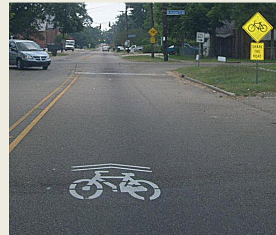
Example of roadway with “Share the Road” signs & “Sharrows”.
