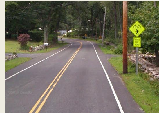
Harvard Road after reconstruction.
