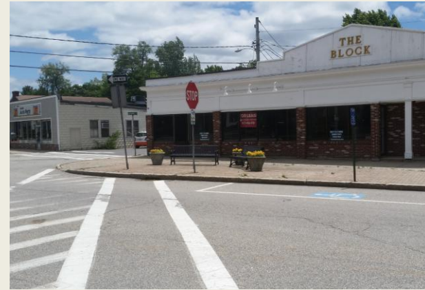
Wide brick buffer between the curb and sidewalk on Stevens St.
