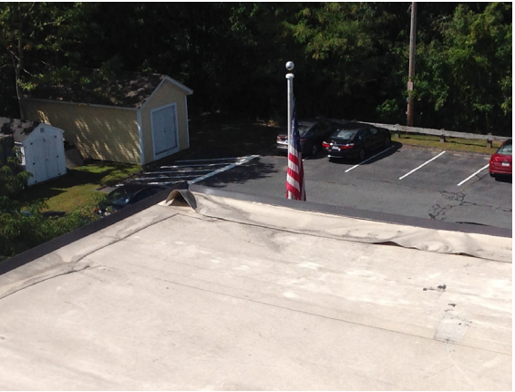
Evidence of water ponding, signs of aged flashings can be seen where membranes seperate, or "pull back". (Classroom Wing- Roof 5)
