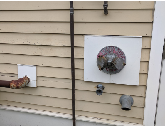
Visible horizontal crack in clapboard siding and trom at pipe penetration.
