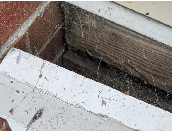
Closeup at horizontal trim board seperation, exposing wall back up.
