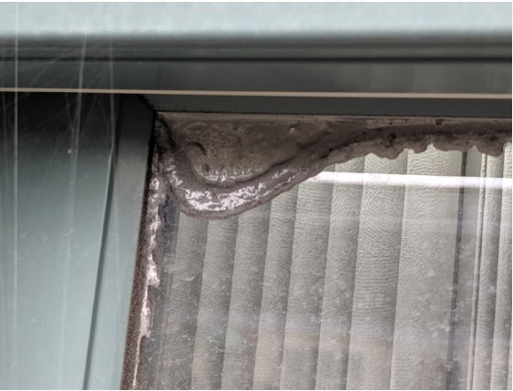
Evidence of sealant failure at sash head.
