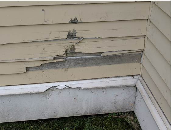
Evidence of missing and damaged clapboard sections, and wood trim.
