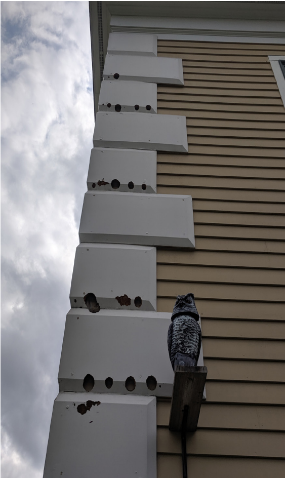
Closeup at damaged painted foam quions from woodpeckers at northeast corner.
