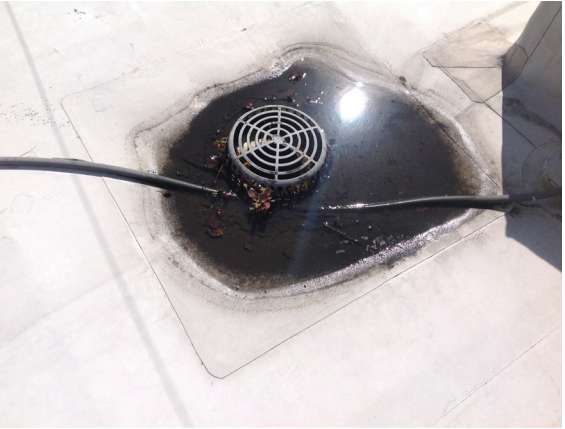
Ponding on roofing at roof drain. (Office Wing - Roof 8)
