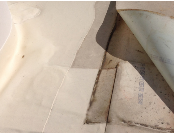
Seperation of an already repaired joint (via applied darker coating) occurring in mansard wall. (Classroom Wing - Roof 5)
