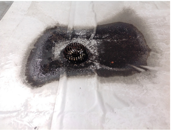
Evidence of ponding of water and debris near roof drain. (Library Wing - Roof 2)
