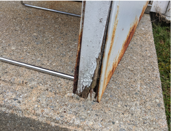
Evidence of damaged & deteriorated paint finish, and rotting (loss) of core material.
