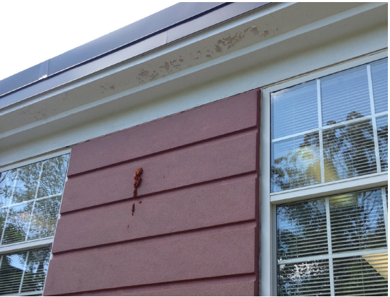
Damage from nesting birds that has been reactively filled with spray foam that does not match finish of Dryvit. (Library Wing - Shattuck Street Side)
