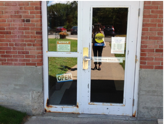
Evidence of damaged & deteriorated paint finish, and rotting (loss) of core material. (Library Wing - Parking Lot Side)
