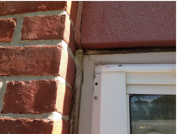
Evidence of cracked caulking at window opening. (Library Wing - Parking Lot Side)
