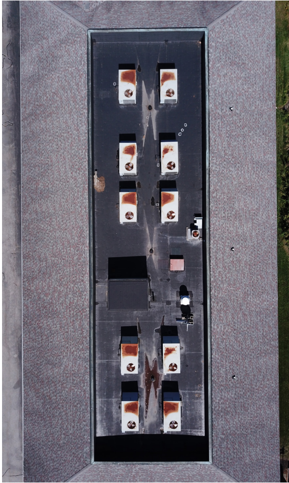
Evidence of deteriorated RTUs in need of replacement.
