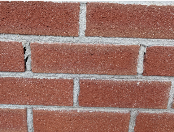
Poorly toothed mortar, seperation can be seen at head joint.
