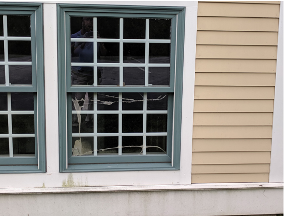
IGU at lower sash broken, should be replaced.
