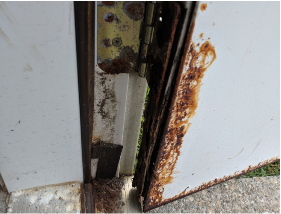
Evidence of damaged & deteriorated paint finish, and rotting core material.
