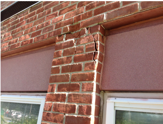
Evidence of brick spalling, most likely from uneven compression and/or water damage. (Library Wing - Parking Lot Side)
