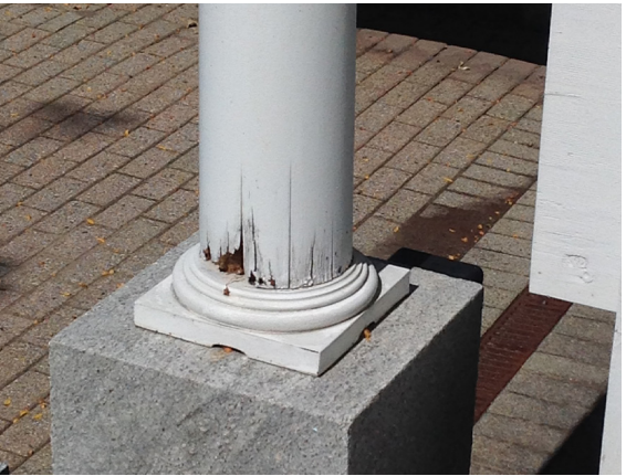
Evidence of cracking/missing wood on column trim. (Library Wing - Parking Lot Side)
