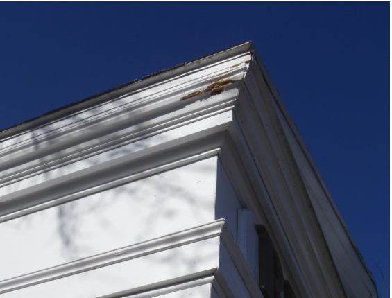
Evidence of damage to trim, most likely from an animal. (Library Wing - Shattuck Street Side)
