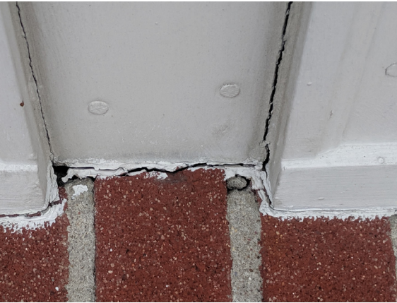
Evidence of missing mortar and lack of sealant, this is a source of potential water infiltration.
