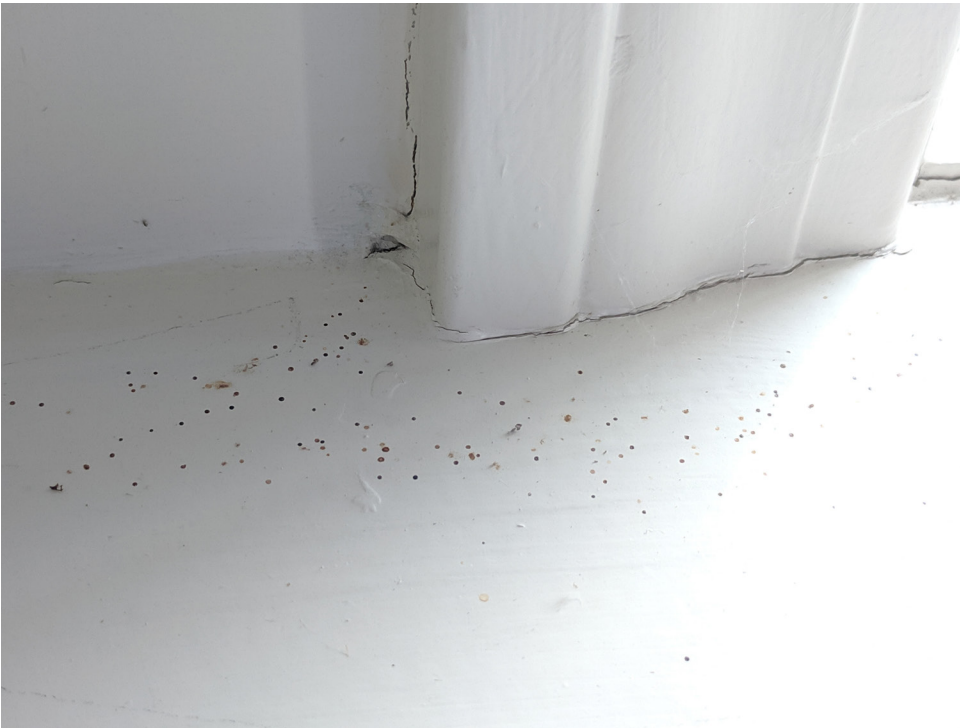
Visible evidence of pest activity at East window sill, first floor.
