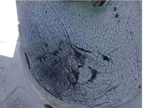
Evidence of cracked roofing membrane, due to moisture damage / ponding of water. (Office Wing - Roof 8)
