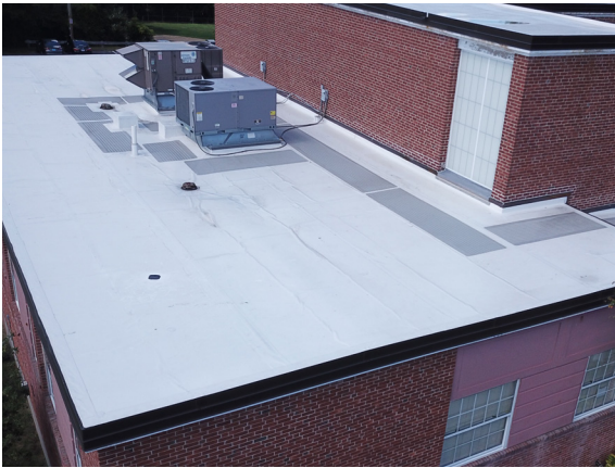
Evidence of rippling at roof membrane seams. (Library Wing - Roof 1)
