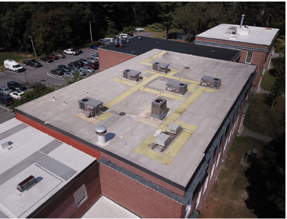
Overall discoloration of roof. (Classroom Wing - Roof 5)
