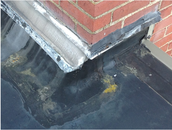
Organic growth around base flashing and gap in flashing near Classroom Wing. (Multi-Use Wing - Roof 6)
