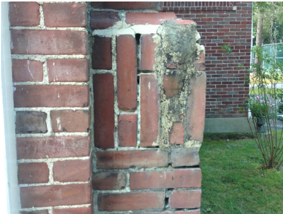
Evidence of attempted patch of corner with mortar and areas of missing mortar. (Office Wing - Shattuck Street Side)
