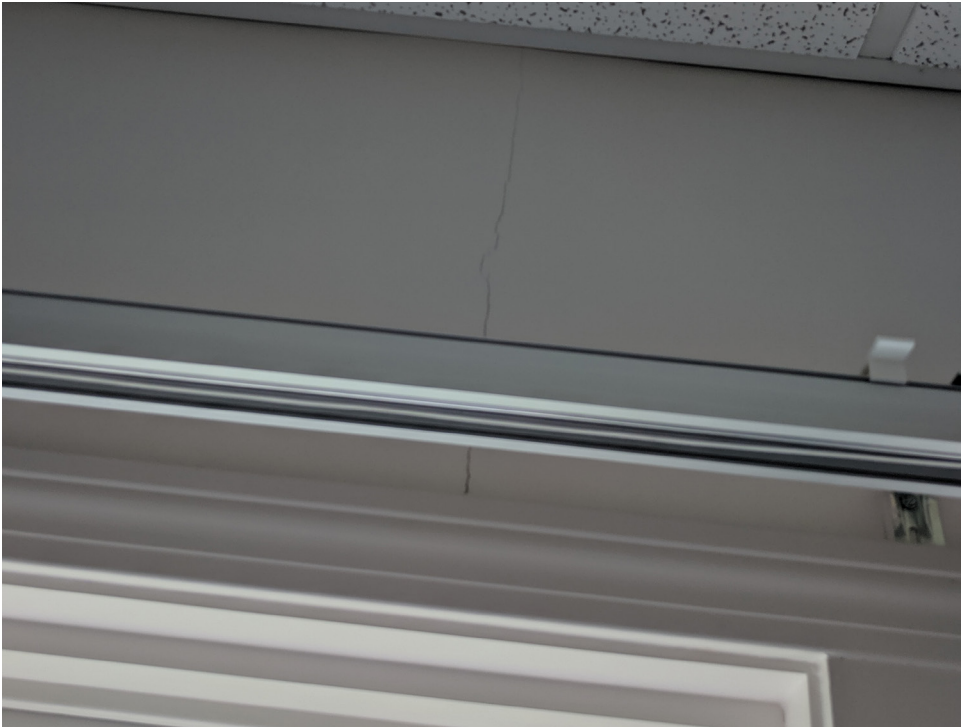
Observed crack above window head, second floor east wall.
