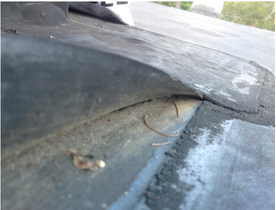
Evidence of water ponding, signs of aged flashings can be seen where membranes seperate, or "pull back". (Multi-Use Wing - Roof 6)
