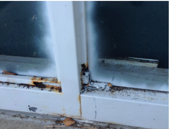
Closeup at of aluminum sidelight sill at library main entrance. (Library Wing - Shattuck Street Side)
