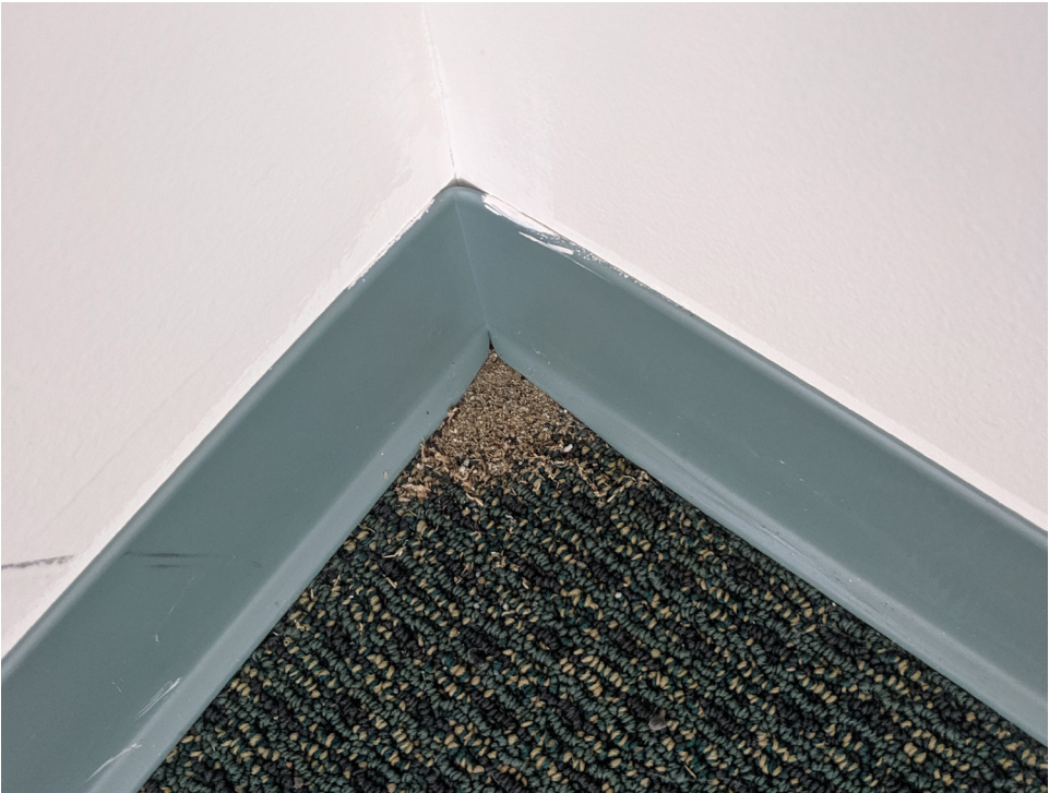
Evidence of what appears to be frass, first floor East corner at wall base corner.
