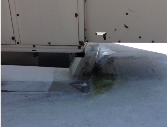
Evidence of ponding of water near mechanical unit. Gap in base flashing. (Office Wing - Roof 8)
