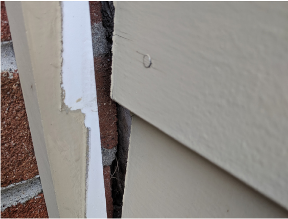
Closeup at vertical trim board seperation, exposing wall back up. We can note that there is no evidence of a sealant joint.
