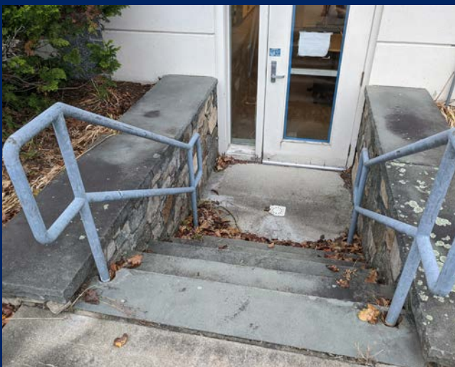
Photograph of the exterior landing and stairs, leaves and lichen should be cleaned regularly.
