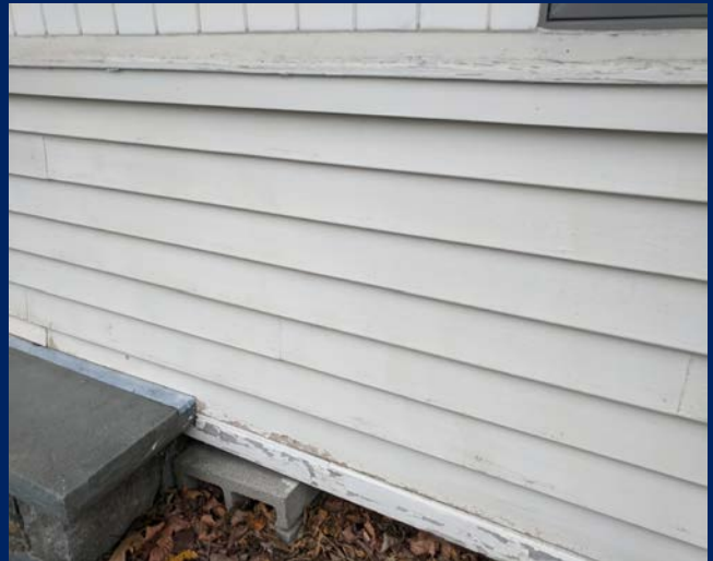
Close up view at a location where paint loss is occurring on the siding.
