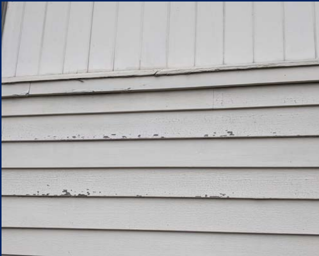
Close up photograph at typical clapboard siding shows signs of paint loss.
