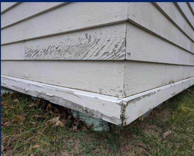
A typical corner condition showing paint loss and amage to trim boards.
