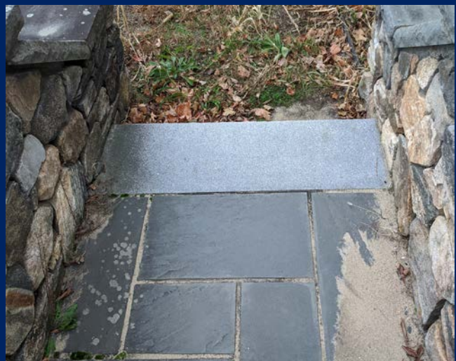
Photograph of the exterior landing and stairs, sand and moss should be cleared regularly.
