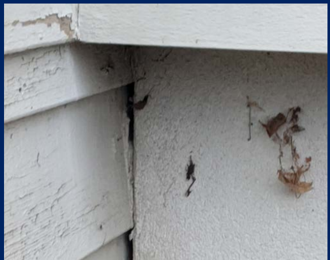
Close up detail where siding meets foundation wall, this joint should be cleaned and sealant applied.
