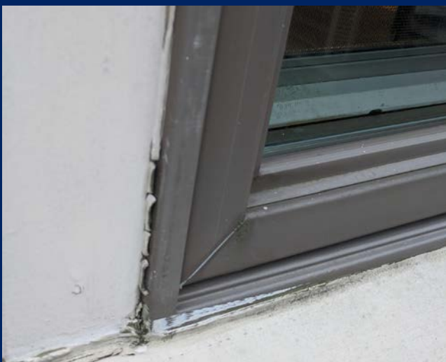
This photograph shows loss of the sealant at the window perimeter as well as some dirt which can be cleaned.
