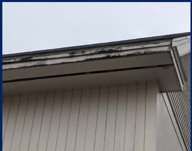
This photograph shows the condition of the roof trim and loss of finish paint exposing the wood substrate.
