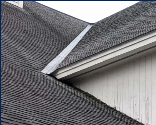
Detail view at valley intersection, vertical wall shows organic growth. Streaking and staining can be observed.
