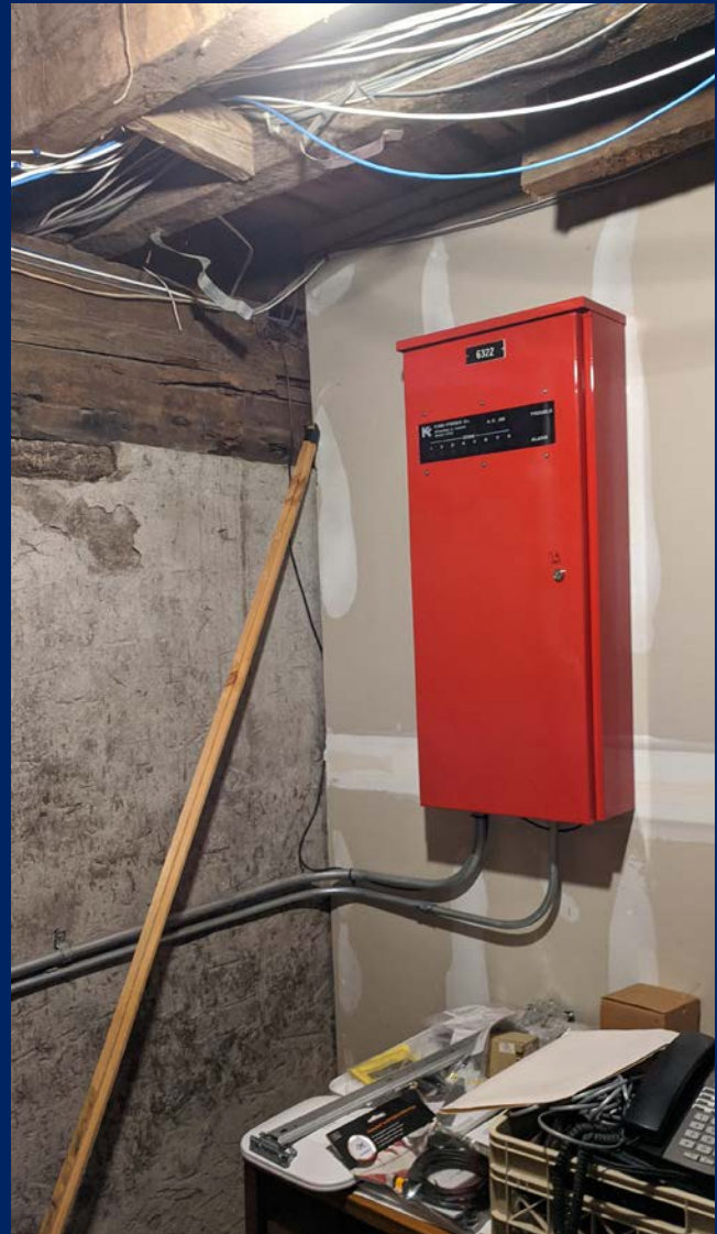
Fire protection system panels. (Basement)
