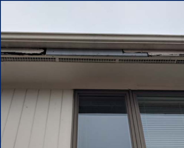
View from the ground at roof soffit where small repair was attempted to enclose lost wood trim. Condition to be monitored.
