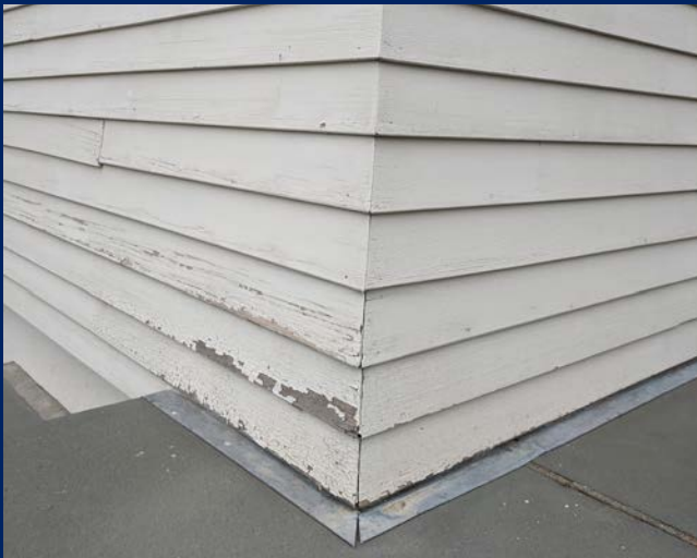
Exterior corner shows paint deterioration and mitred joints that have begun to separate.
