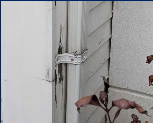
Water damaged trim board at gutter bracket, paint loss and trim should be repaired to prevent further damage.
