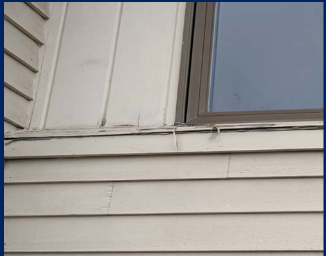
Close up view of trim transition condition where paint finish is beginning to fail.
