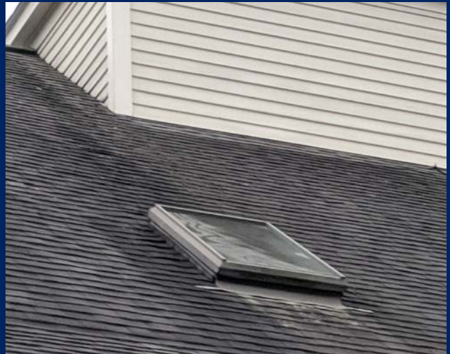
Streaking and staining can be observed at one of the skylights on the north roof.
