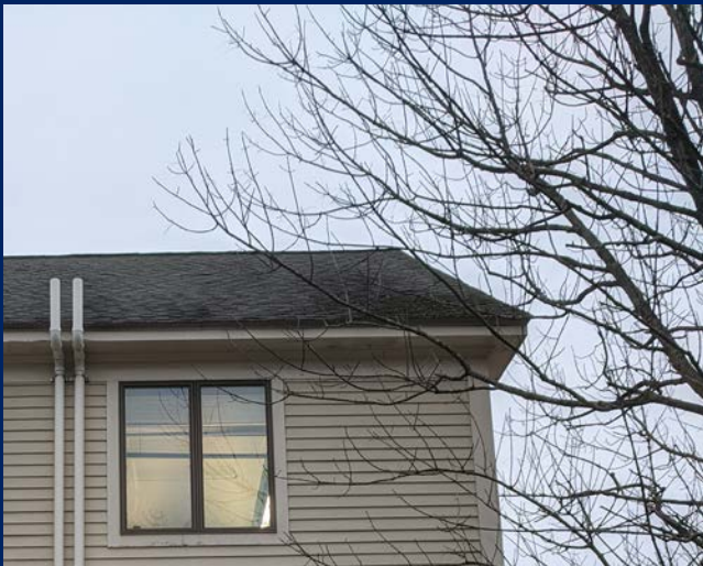
Abrasive wearing can be observed at the SW corner under the tree canopy.
