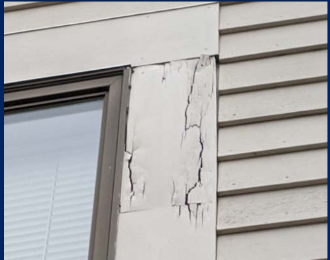
Close up view of failing paint finish and potentially damaged wood substrate.
