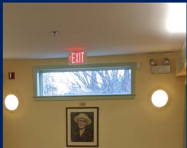
Typical Fire Alarm (strobe/alarms, exit signs and emergency lights) and Sprinklers throughout corridors and offices. (Second Floor)
