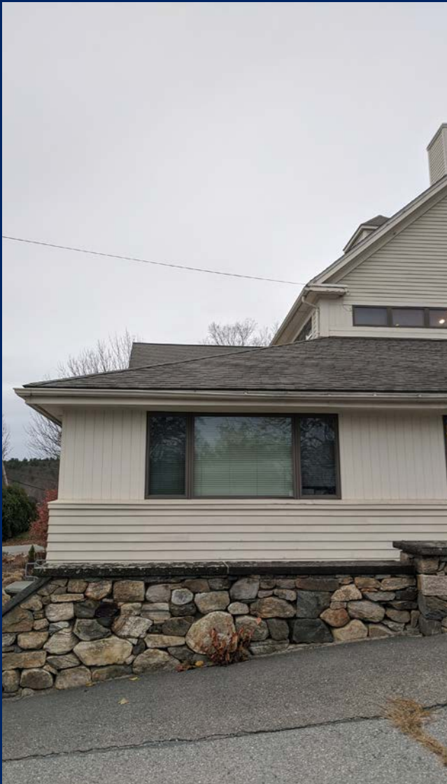
View of exterior wall, plant growth at base and on wall should be removed.
