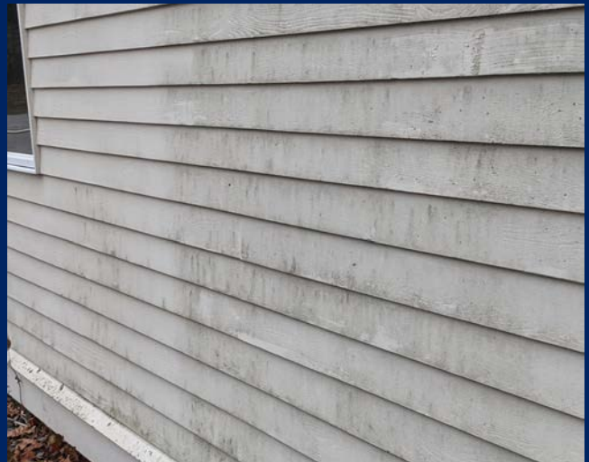
Generally the exterior siding should be cleaned to remove organic growth.
