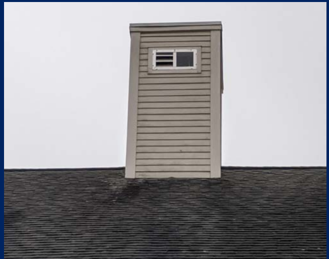
Detail view at chimney. Streaking and staining can be observed.
