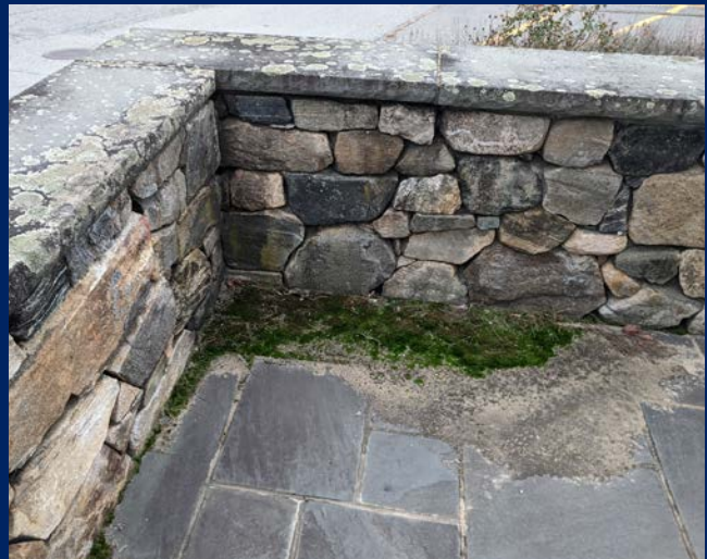
Photograph of the exterior landing, sand and moss should be cleared regularly.
