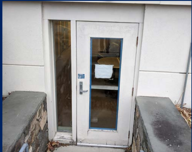
This door and frame from the basement are reaching the end of useful life and should be replaced with an FRP door and frame.
