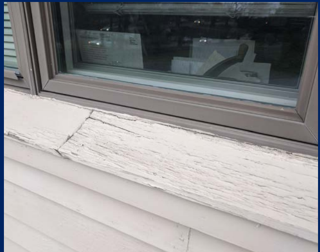
View of a typical window sill, generally the window is in good condition, the wood trim however needs to be addressed.
