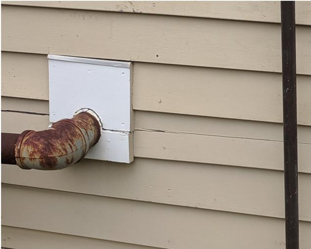
Visible horizontal crack in clapboard siding and trim at pipe penetration.
