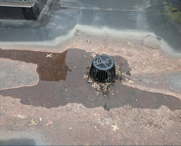
Ponding on roofing at roof drain.
