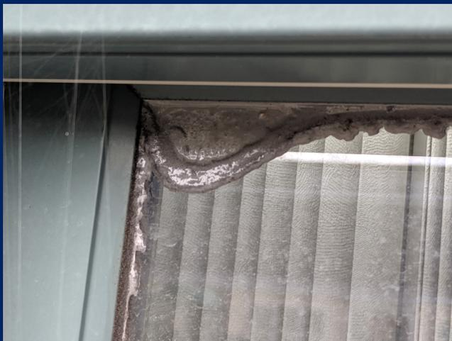
Evidence of sealant failure at sash head.
