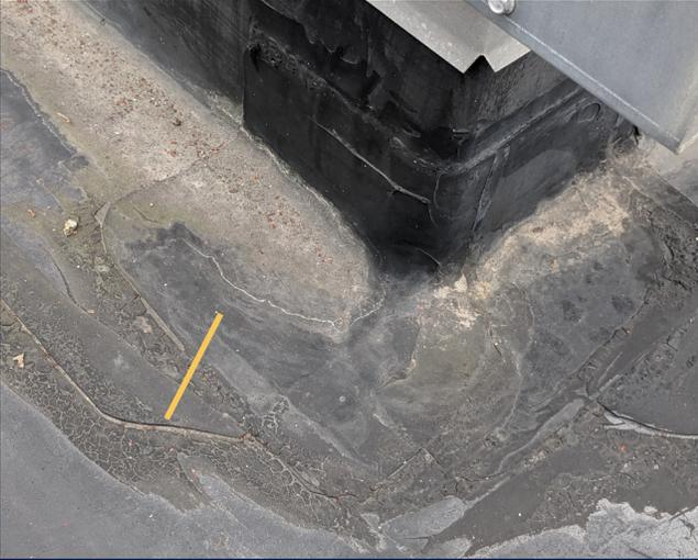
Evidence of water ponding, signs of aged flashings can be seen where membranes separate, or "pull back".
