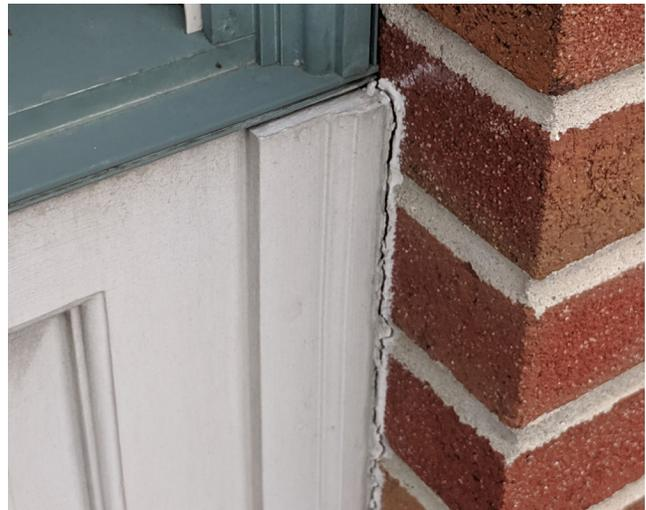
Closeup at vertical trim board at window infill panel. Note separation of a sealant joint at brick.
