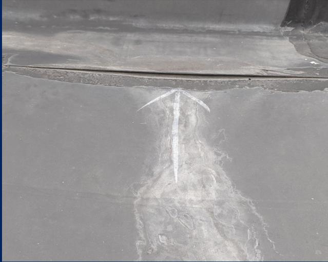
Evidence of ponding of water near mechanical unit. Gap in base flashing, chalk arrow (placed by others) points toward gap.
