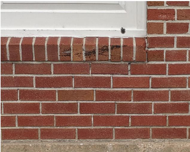
It appears as though the building sustained vehicular impact, you can see crack lines in the mortar.
