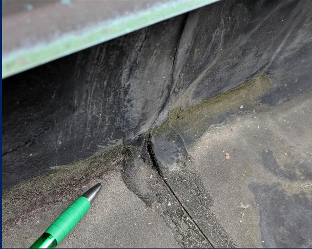
Organic growth around base flashing and gap in flashing.
