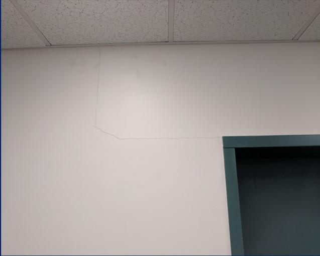
Observed crack above elevator door head, second floor.
