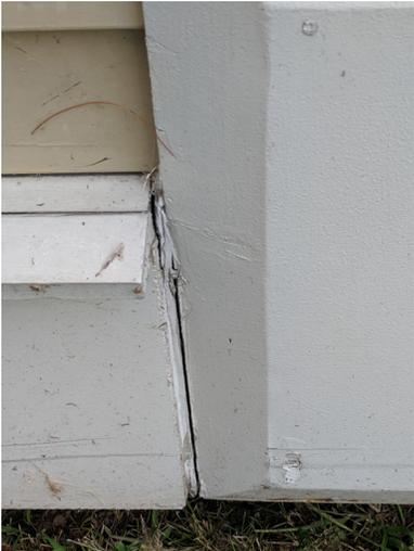
Closeup at horizontal trim board end abutting quion. Note sealant joint has failed and is separated.
