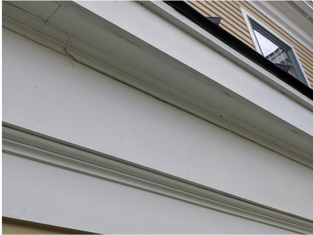
Observed horizontal cracked eave trim. Note, you can follow the crack from the upper edge, through the trim, to the bottom.
