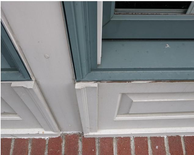
Closeup at top of window infill panel, note advanced weathering of unflashed horizontal edge (R), as well as lack of sill flashing.
