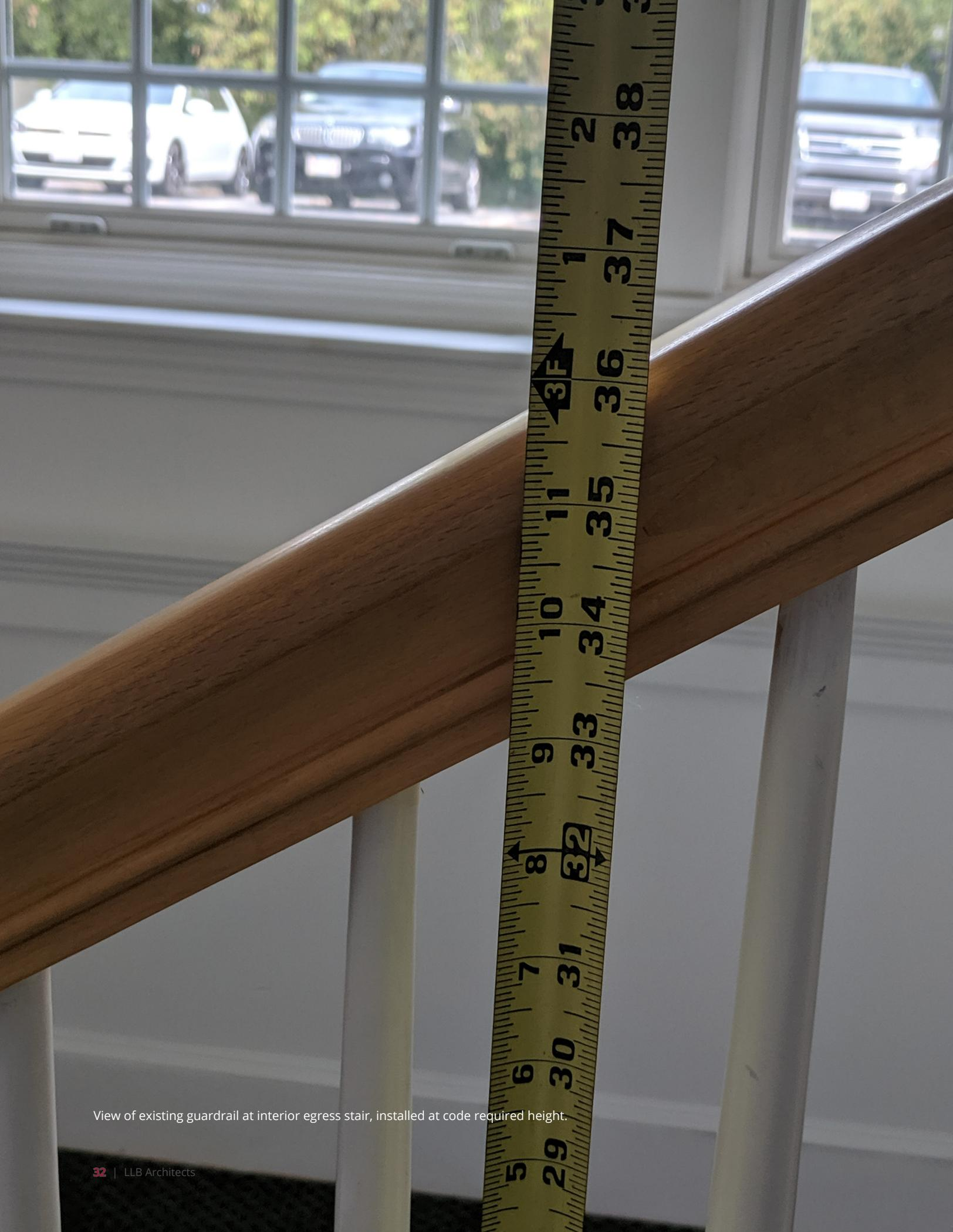
View of existing guardrail at interior egress stair, installed at code required height.
