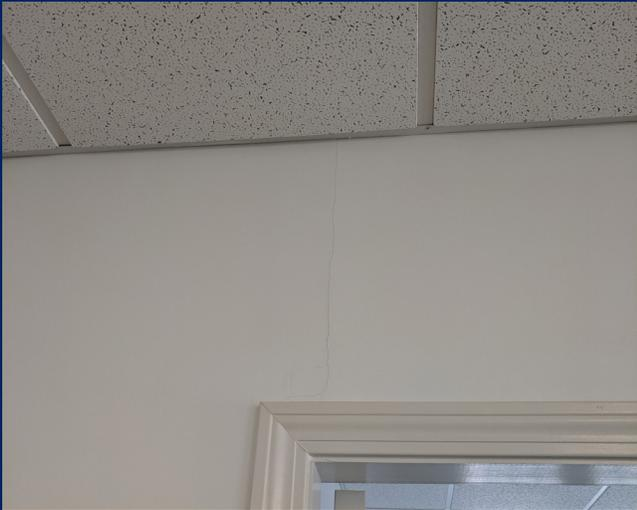
Observed crack at interior wall above door, first floor north.
