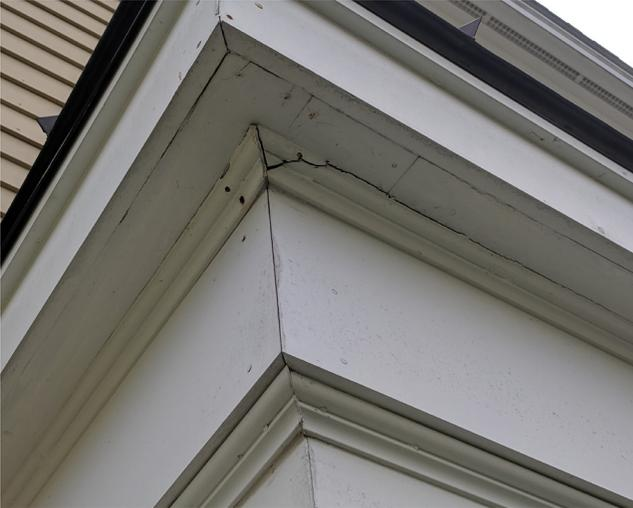
Observed horizontal cracked eave trim at corner, appears to start at mid trim and travels horizontally at upper edge.
