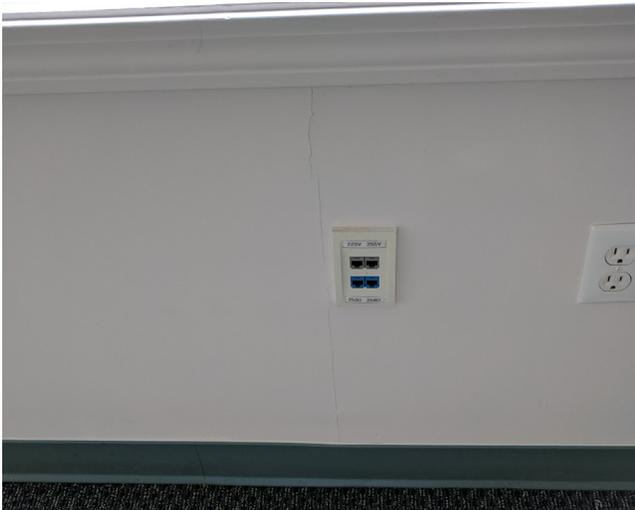
Observed crack below window sill, second floor east wall.
