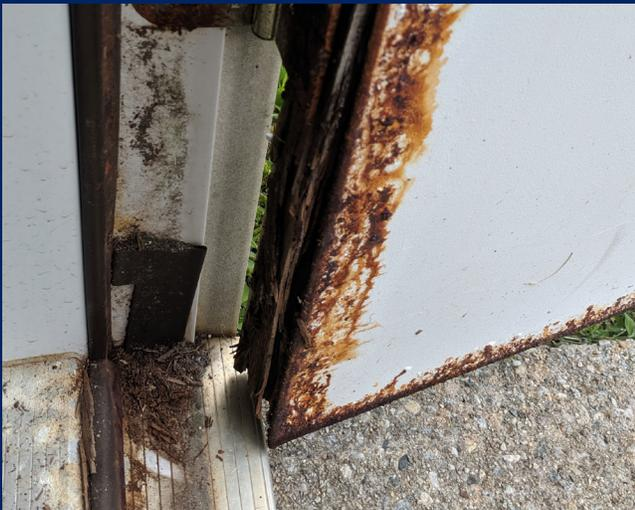
Evidence of damaged & deteriorated paint finish, and rotting core material.
