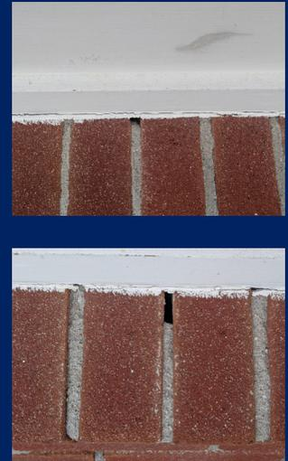
Various points of missing mortar at the exterior sills.
