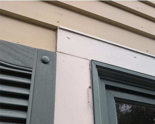
Closeup at vertical window trim board. Note sealant (or paint) failure at frame.
