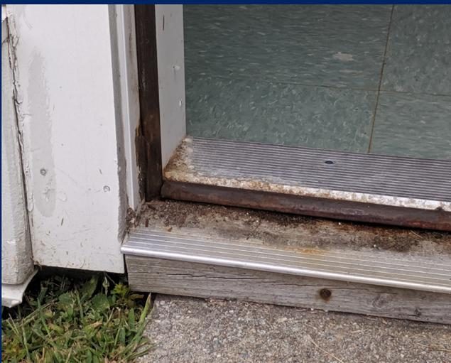
Evidence of damaged and rusting sill.
