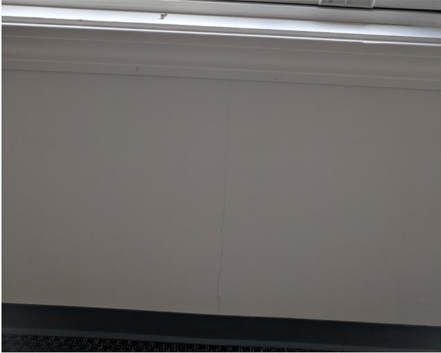
Closeup at bottom of window showing crack, second floor, east exterior wall.
