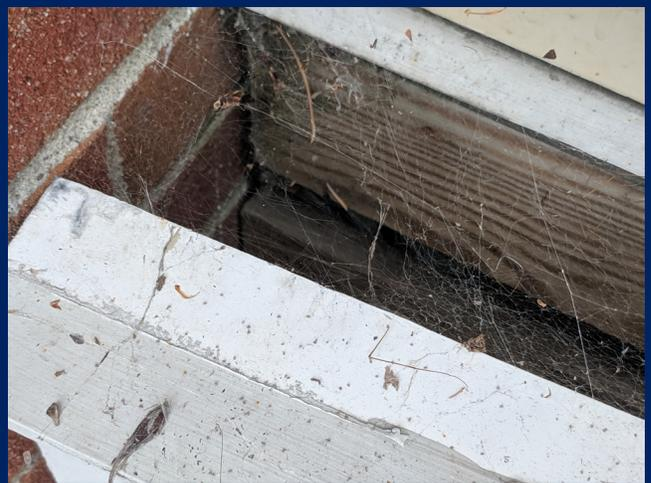
Closeup at horizontal trim board separation, exposing wall back up.
