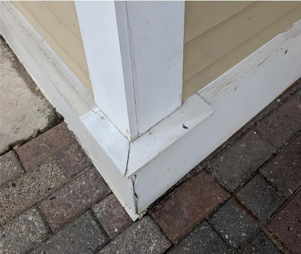
Observed horizontal wall trim board separated at corner.
