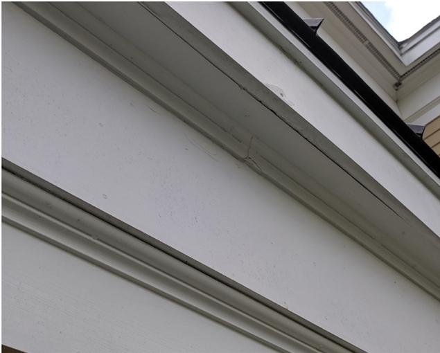
Observed cracked eave trim. Note, you can follow the crack from the upper edge, through the trim, to the bottom. Also you can see the bowed vertical fascia creating a gap.
