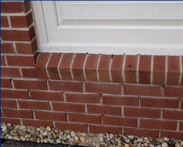
Visible mortar missing at window sill, and poor toothing of joints on vertical surface joints, lack of weeps low on the wall.
