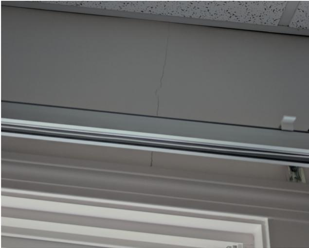
Observed crack above window head, second floor east wall.
