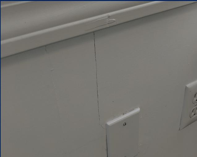
Observed crack at exterior wall below window, first floor east.
