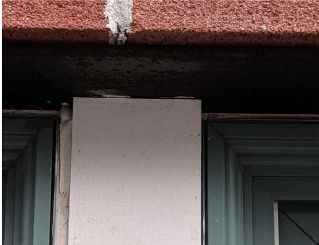
Closeup at vertical trim board between windows, note separation of sealant (L), no evidence of a sealant joint (R).
