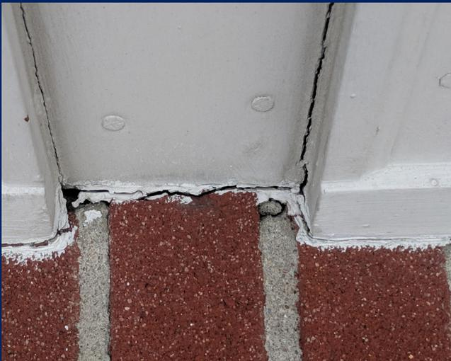
Evidence of missing mortar and lack of sealant, this is a source of potential water infiltration. .
