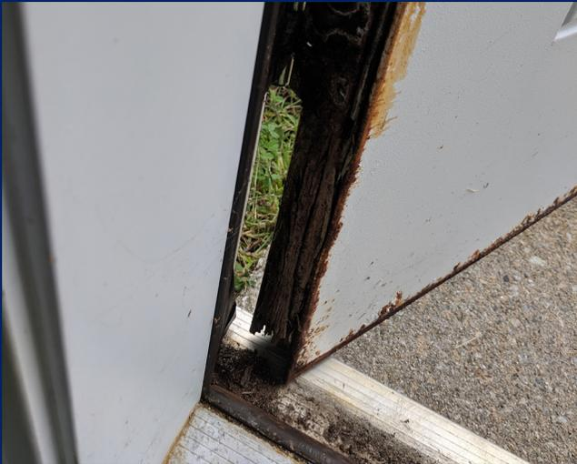
Evidence of damaged & deteriorated paint finish, and rotting (loss) of core material.
