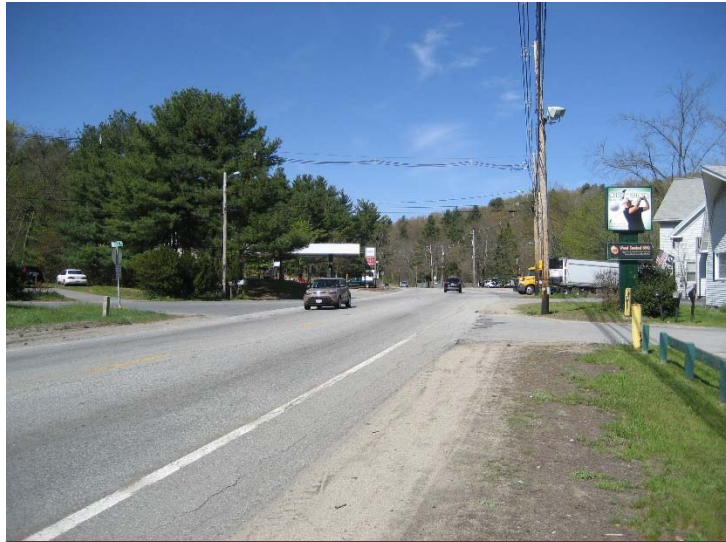
Route 2A/110, looking west towards the unsignalized intersection with Willow Road/Bruce Street
