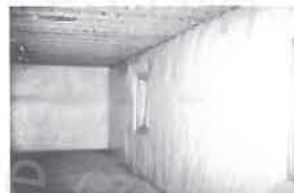
Photograph 3 Blanket insulation with impermeable vinyl interior surface
