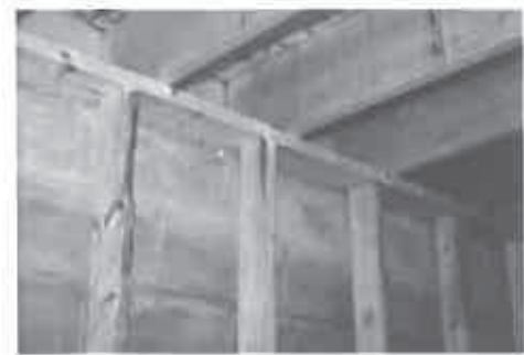
Photograph 1 Interior stud framing located at basement perimeter
