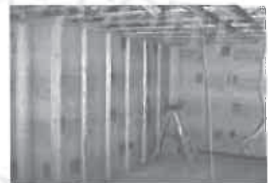
Photograph 8 Unfaced extruded polystyrene against basement wall
