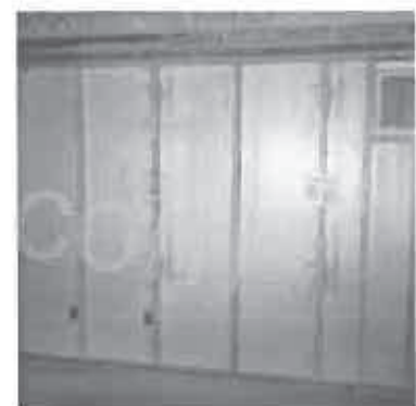
Photograph 9 Unfaced extruded polystyrene against basement wall
