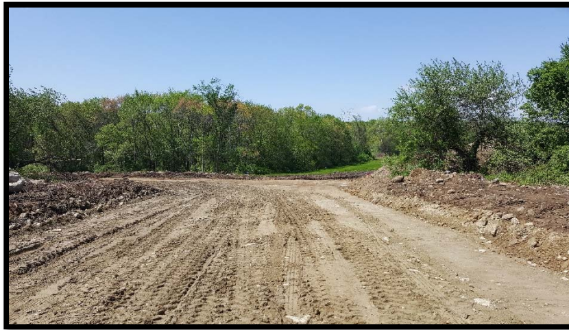
(Standing on Couper Farm Lane Sta. 2+00, looking west)
