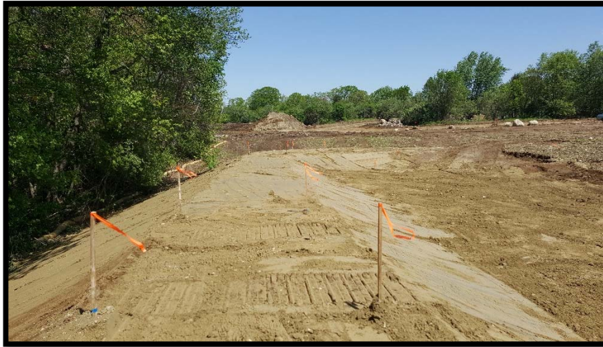
(Standing on the berm for Infiltration Basin No. 2, looking north)
