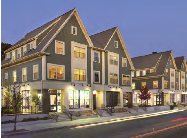
Tall peaked roofs reduce the apparent scale of these mixed-use blocks while accommodating a full third floor. Highly transparent windows and doors on the ground floor are critical to maintaining a lively pedestrian environment (Courtesy Union Studio, Architects)
