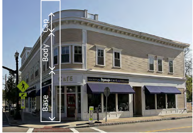
A time-tested design for a “Main Street” block in Holliston, MA, with shops on the ground floor and apartments or offices above. Awnings control glare and heat while allowing for large, transparent windows on the ground floor. The traditional design of “base, middle and cap” provides for attractive proportions.
