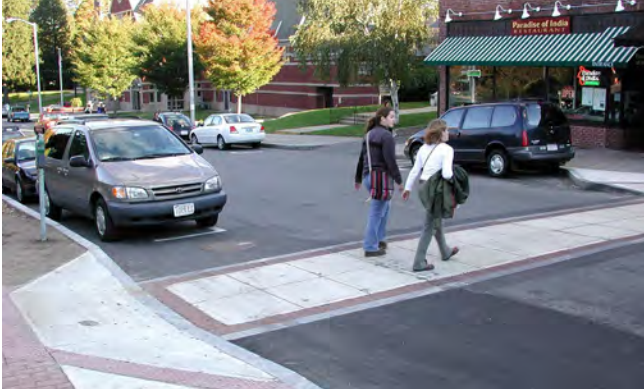
Crosswalks should feature a change of materials and texture to enhance visibility. Durable stone, brick or concrete help to tie crosswalks into the larger pedestrian system, and hold up better than paint.
