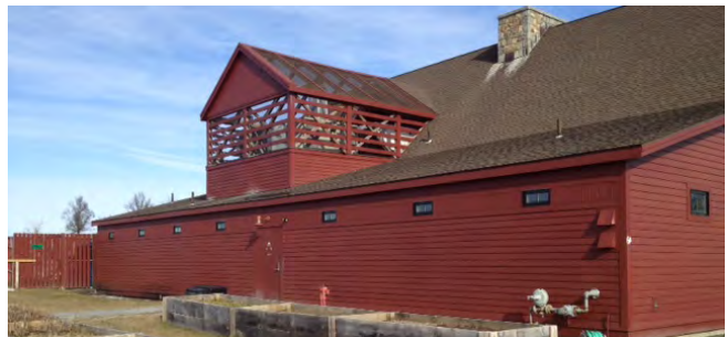
Service areas and mechanical equipment should be screened and screening elements incorporated into the architecture.
