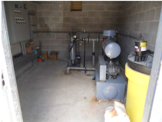
Photo #39: Septic system pump equipment
