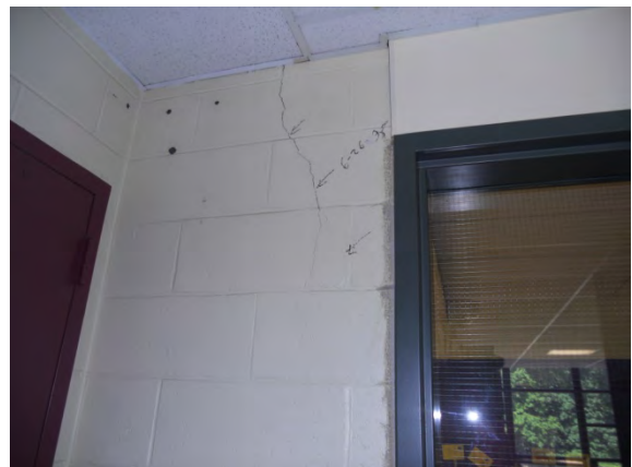
Photo #42: Settlement cracking at second floor of stairwell adjacent to generator room
