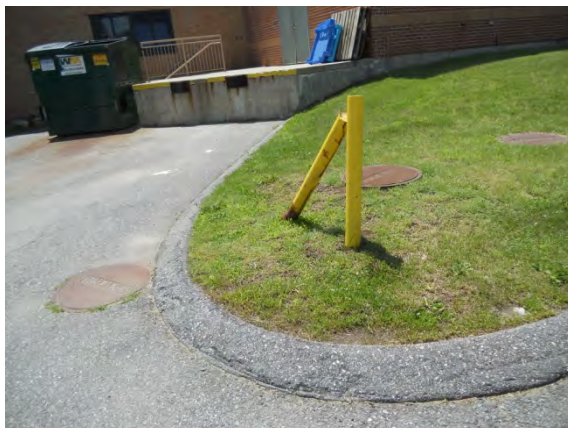
Photo #41: Loading dock with damaged bollards
