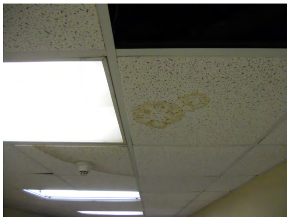
Photo #25: Water staining
