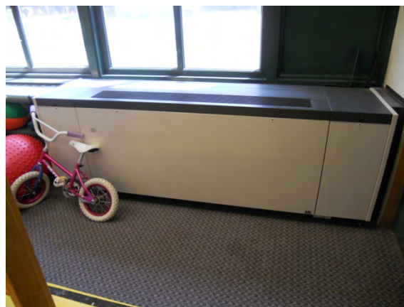
Photo #30: New univentilator
