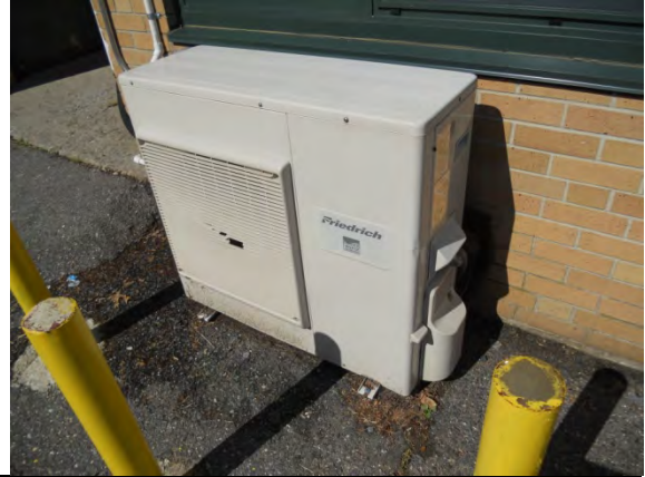
Photo #50: Ductless mini-split air conditioner
