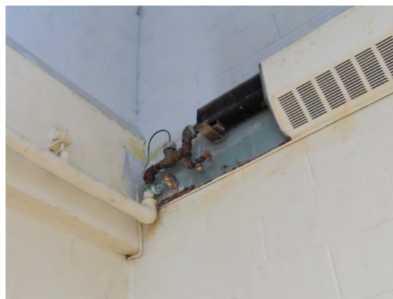
Photo #24: Wall mounted radiant heater with missing cover
