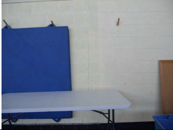
Photo #43: Cracking in gymnasium
