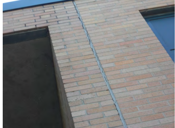
Photo #14: Deteriorated expansion joint
