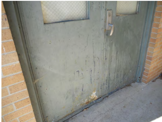
Photo #51: Rusty and deteriorated service door
