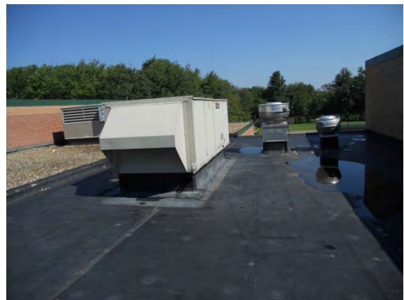
Photo #54: Rooftop makeup air handling unit with rooftop unit behind to the left and exhaust fans to right
