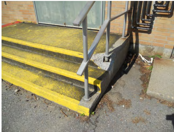
Photo #15: Deteriorated concrete at rear steps
