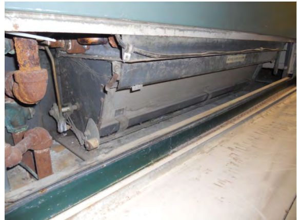
Photo #34: Older univentilator piping and grill
