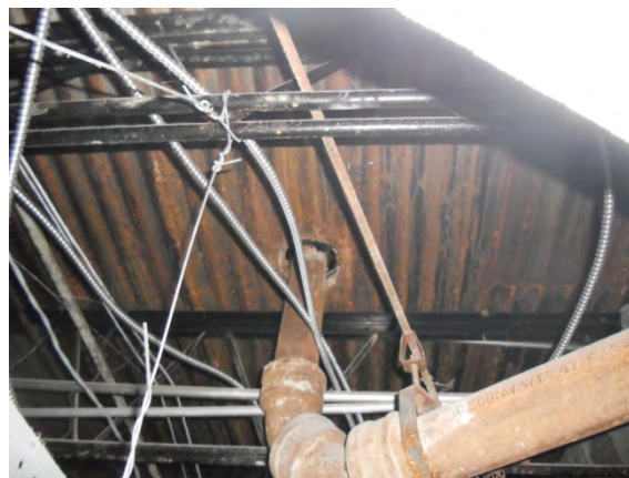
Photo #26: Drain line above stained ceiling tiles
