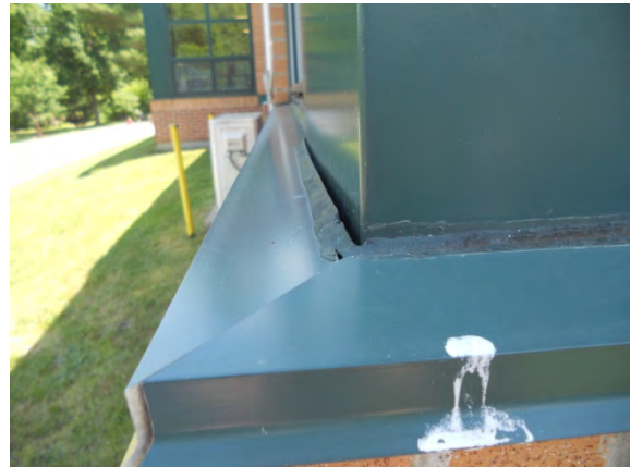
Photo #40: Deteriorated sealant at rear of building at kindergarten classroom addition
