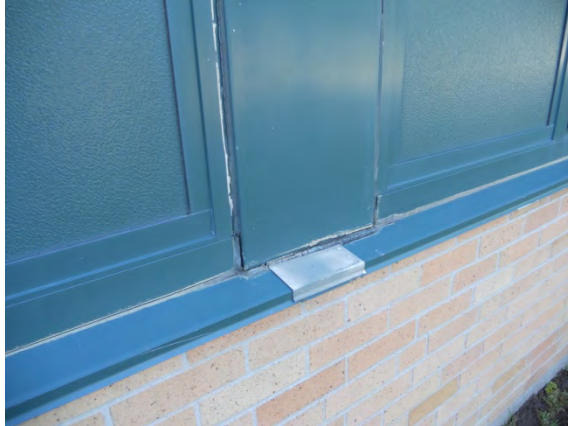
Photo #13: Deteriorated sealant at spandrel panels
