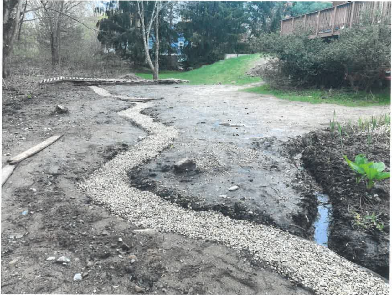
Photo 13. Fill and river rock walkway in BVW
