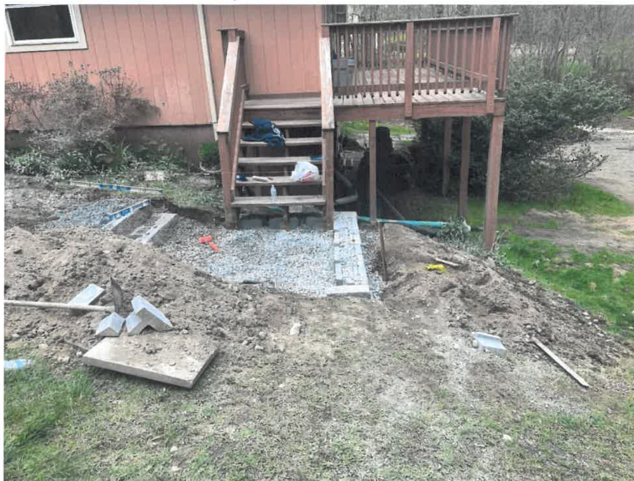
Photo 4. Construction of pavers/gravel walkway and excavated soil
