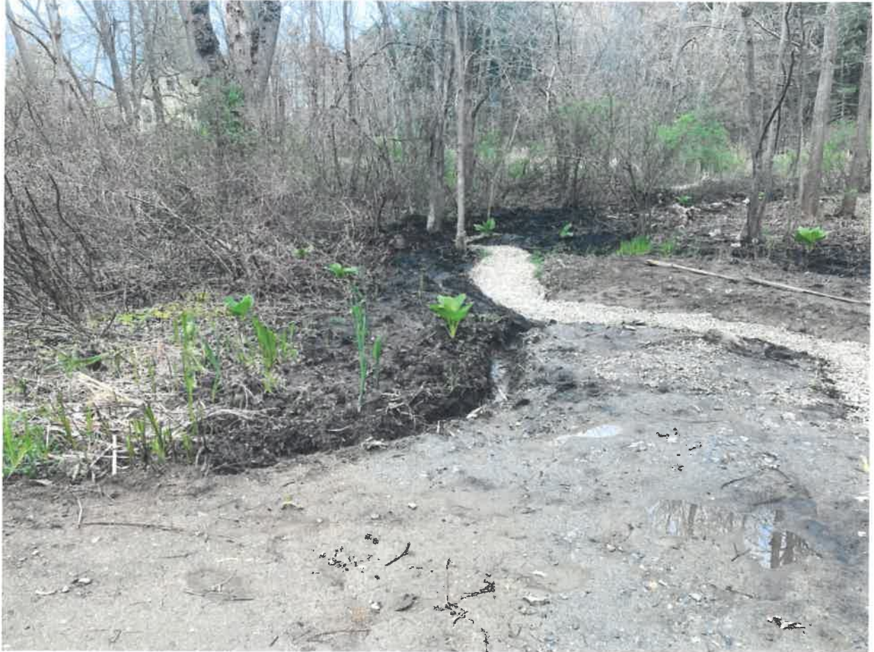
Photo 11. Fill and river rock walkway in BVW
