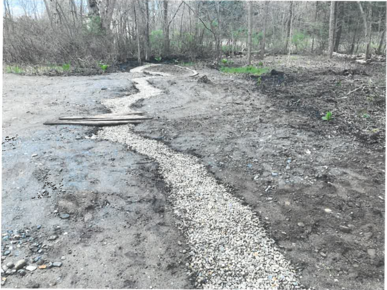
Photo 12. Fill and river rock walkway in BVW
