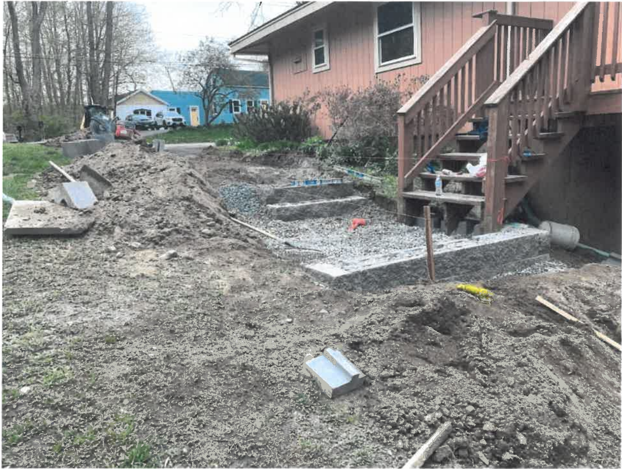
Photo 2. Construction of pavers/gravel walkway and excavated soil
