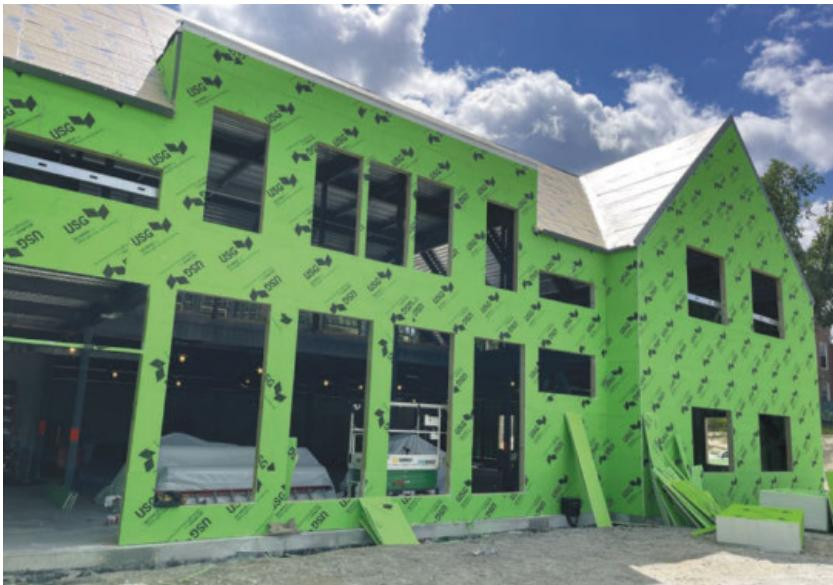
The exterior makes significant progress as the dens-glass gypsum fiber sheathing goes up (the green sheet boards.) The next step is for the waterproofer to seal the joints between the sheets and spray Air Vapor Barrier over the outside of the building.
