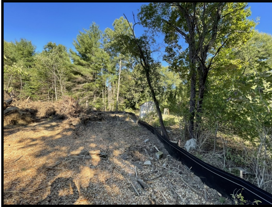
Photo 3: Erosion and sedimentation controls along the northeast site boundary.
