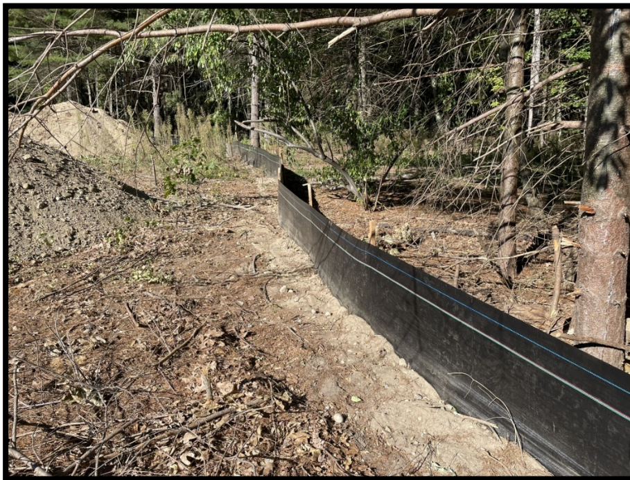
Photo 4: Erosion and sedimentation controls along the northwest site boundary.
