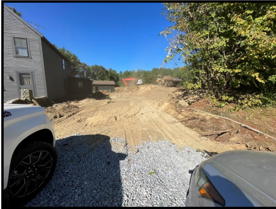
Photo 1 Gravel construction entrance and temporary access corridor.
