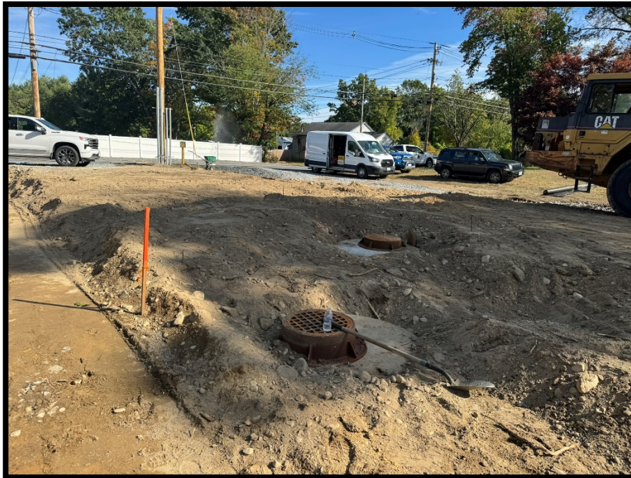
Photo 5: Installed AD-1 & DMH-1
