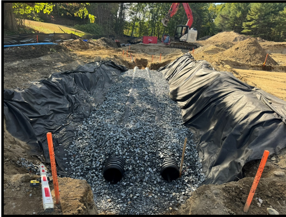
Photo 1: (2) 12 Inch Perforated drainpipes for proposed infiltration basins.
