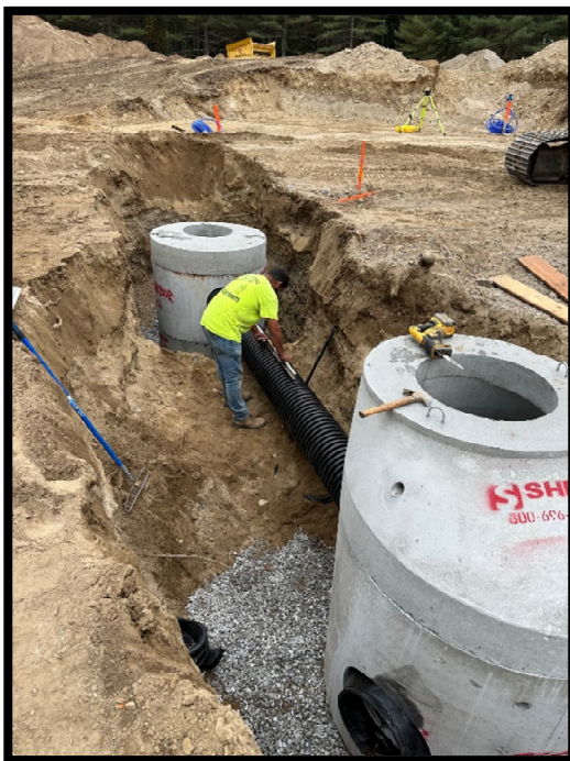
Photo 9 & 10 by MG: DMH-2 and AD-2 Installation
