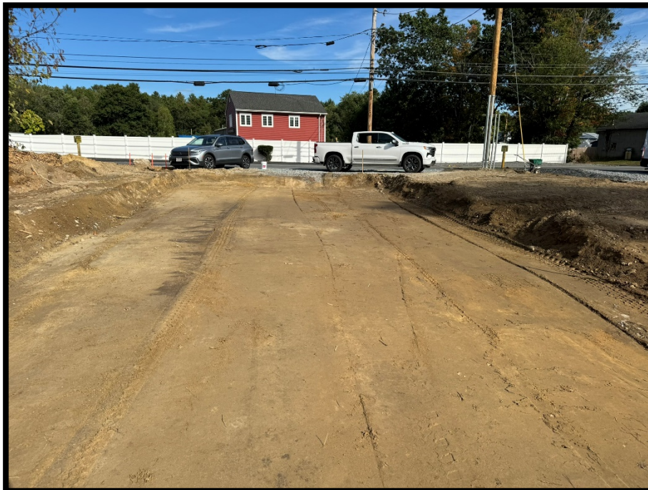
Photo 6: Prepared Subgrade for the Strawberry Farm Road.
