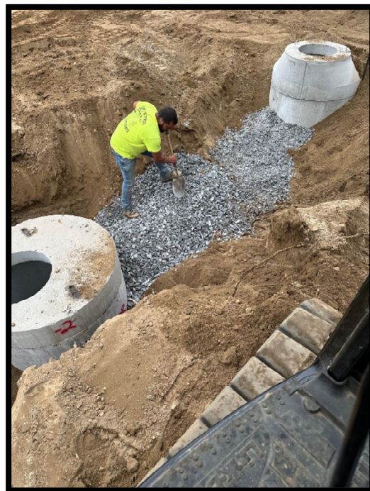
Photo 9 & 10 by MG: DMH-2 and AD-2 Installation
