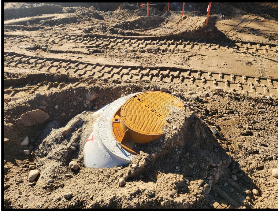
Photo 3: Sewer cover at drain manhole
