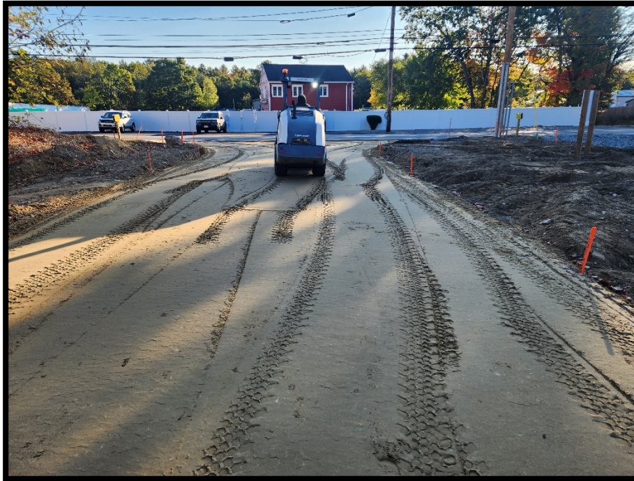
Photo 1: Compaction of gravel subbase continued
