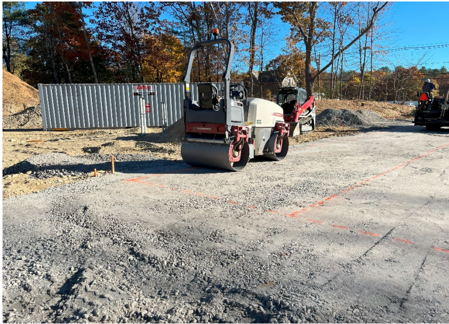
Photo 1: Compaction of gravel subbase
