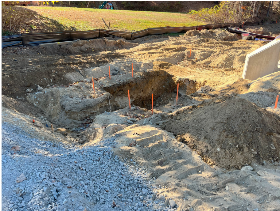
Photo 4: Initial grading at infiltration basin
