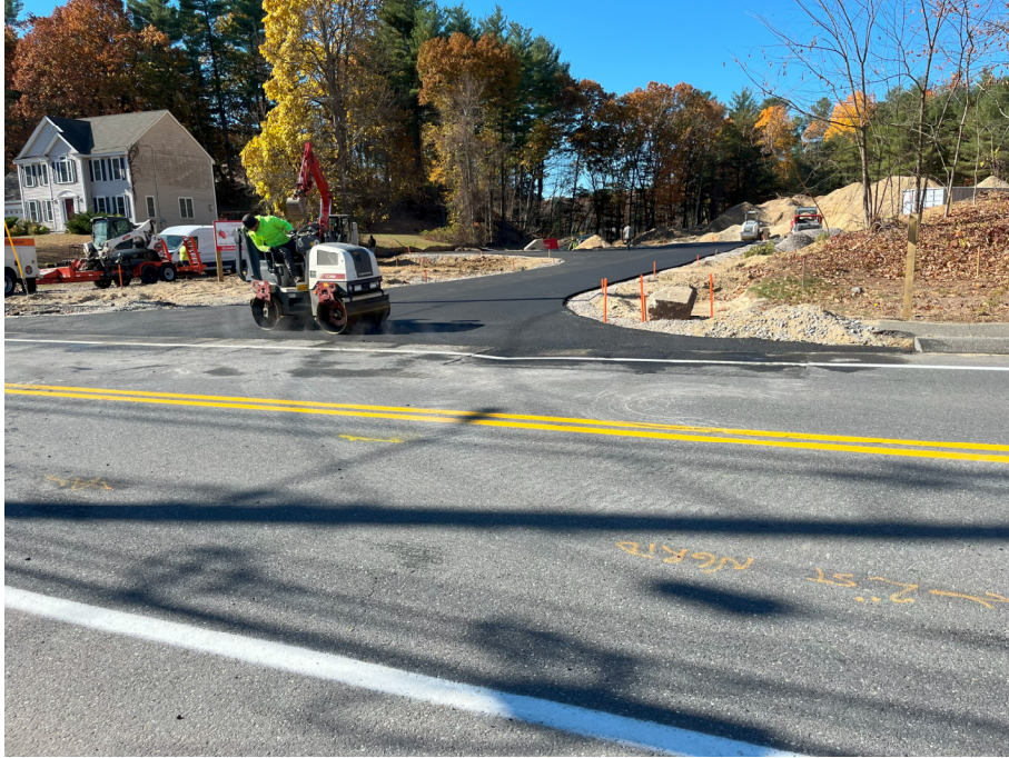
Photo 3: Completed intermediate course placement
