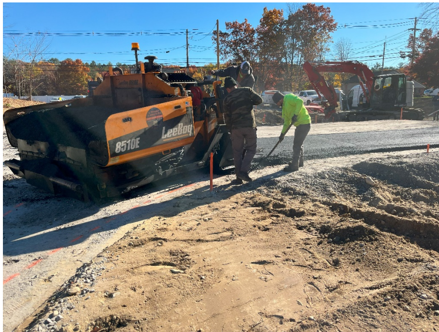
Photo 2: Paving shared driveway
