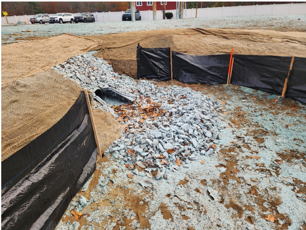
Photo 4: Flared end and check dam at east infiltration basin
