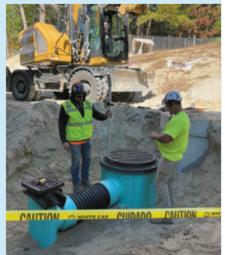
Stormwater drain and catch basin installed and backfilled
