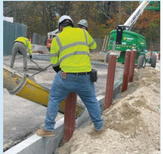
Granite curb and bollards installed
