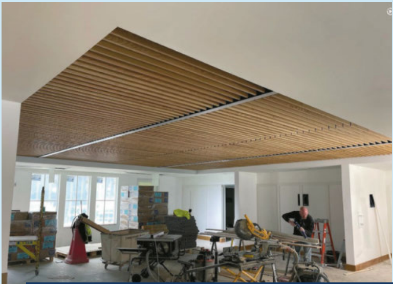
Acoustic ceiling installation in the billiards room
